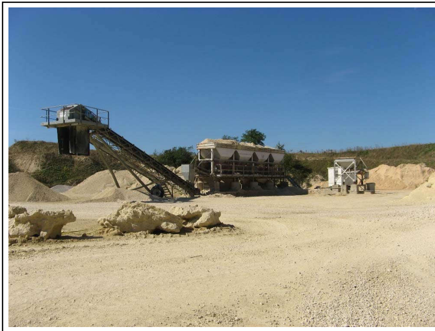
installation de reconstitution.
